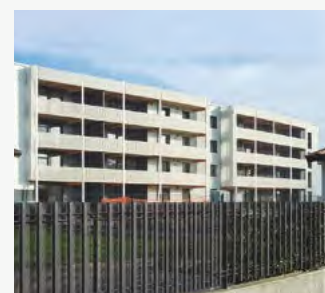
Crosslight House. Residential building. Mulazzano, Italy. PACi and nanoe™ X.
